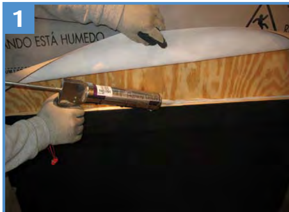
Apply bead of sealant at base of wall.
