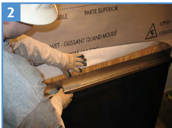
Bed vented starter SSZ-1 into sealant. Overlap SSZ-1 with ZINC PLUS UNDERLAY.
