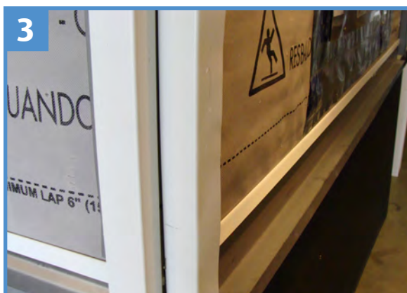
Install VM ZINC PLUS Z flashing WF-H-1 and secure in place with VM ZINC Flatlock clips 16" on center.
