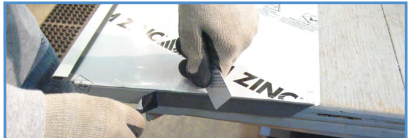
Installation Detail for Jamb Flashing
