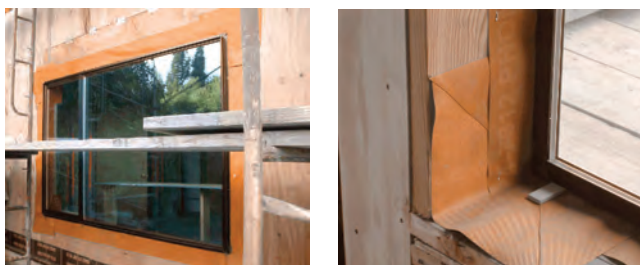
Nail Flange window with VaproFlashing and unique 3D Factory Formed Corners
