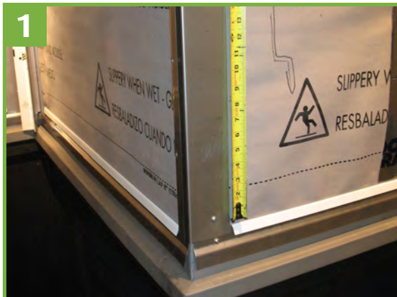
1 Attach pre-punched panel receiver OSC-2 at outside corner.*
