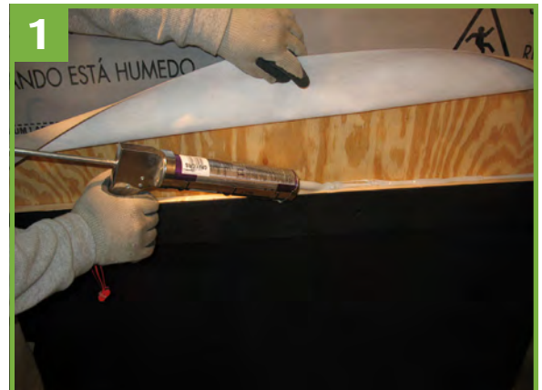
Apply bead of sealant at base of wall.
