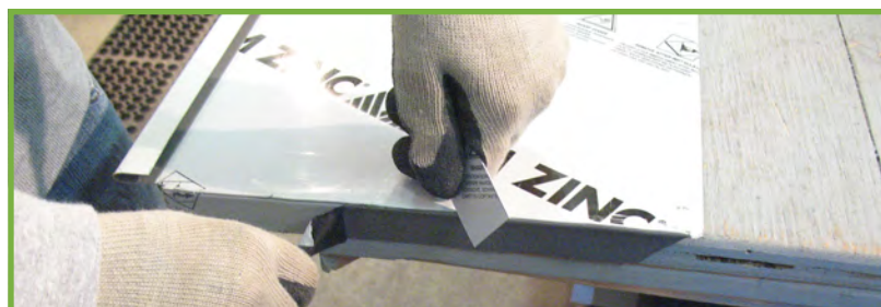
Installation Detail for Jamb Flashing
