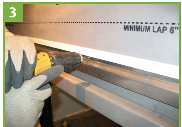
Install VM ZINC PLUS® Z flashing WF-H-1 and off-set starter ST-1. Attach with stainless steel pan head screws.*
