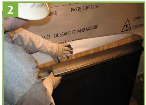
Bed vented starter SSZ-1 into sealant.
