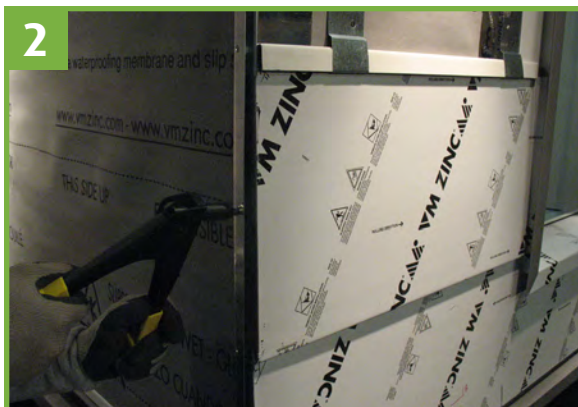
2 Bend end run orientation panels 90 degrees at corner. Fasten inside receiver with stainless steel pop-rivets.
