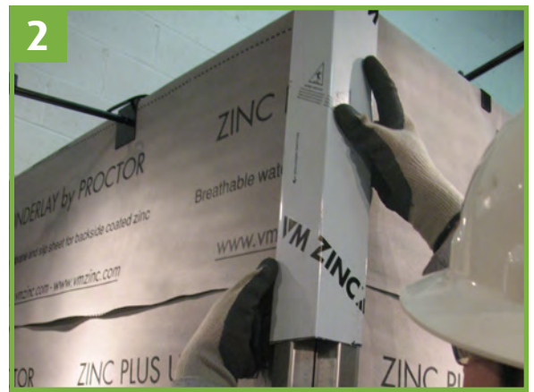
Slide on VM ZINC® PLUS outside corner OSC-1 (shown with masking film attached)
