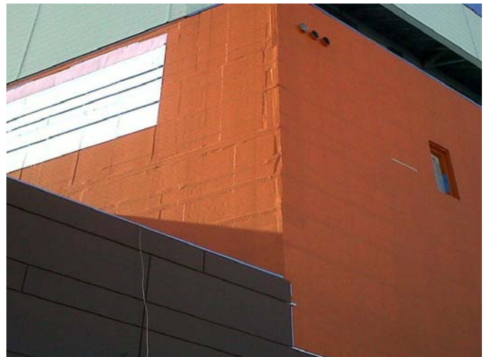
Close up of WrapShield SA Self-Adhered (orange). Note: the tight adhesion to the foam panels (white).
