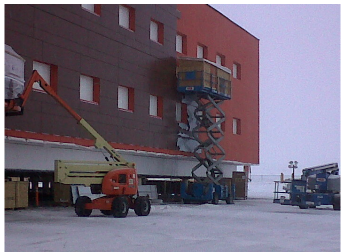
Installation of cladding over WrapShield SA Self-Adhered (orange)
